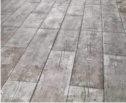
Enhanced Concrete Sidewalk- Stamped and Coloured Wood Texture
