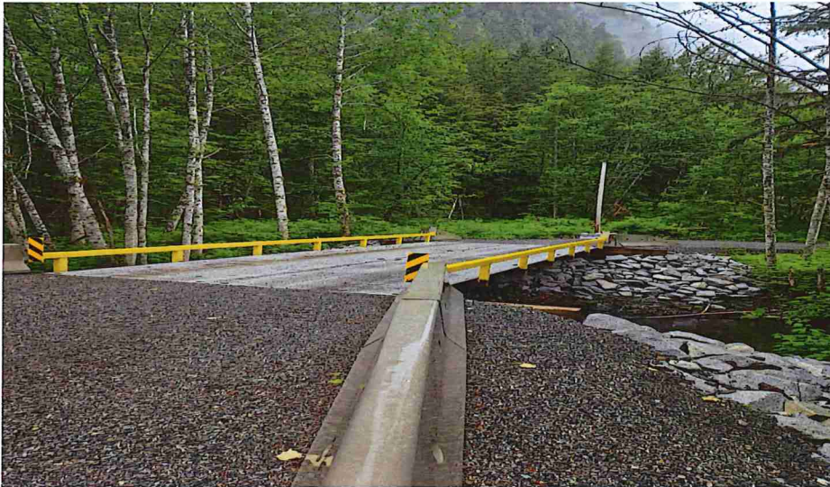
North Rainey Creek Bridge
