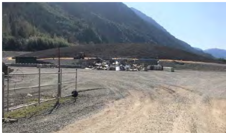
View of the Transfer Station & Landfill Closure
