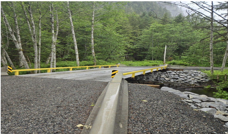
North Rainey Creek Bridge
