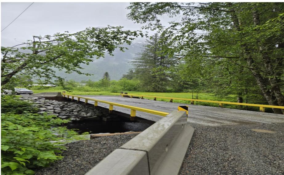
South Rainey Creek Bridge
