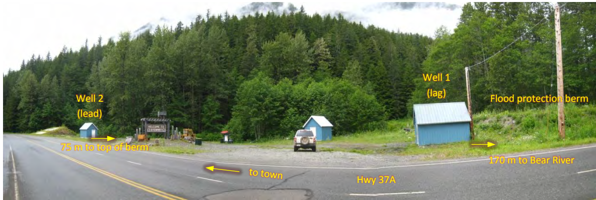
Figure 8. Wells 1 and 2 at north entrance to Stewart.
