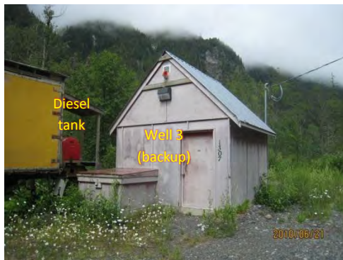
Figure 9. Well 3 at the north end of Brightwell St.
